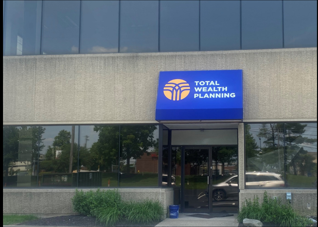
NEW ENTRANCE AT SIDE OF THE BUILDING
